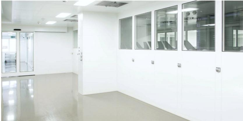
The variety of material types is great: mild steel, stainless steel, galvanized steel and color-coated sheets are available in a colorful mix, depending on the design of the clean room and the visual requests of the customers. The material thickness used for the sandwich wall and ceiling panels is usually 1 mm. Due to the part sizes, which can reach up to 4000 mm long and 1200 mm wide, the folding technology is perfectly suitable.
