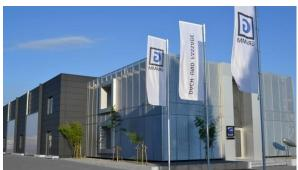
Prokurist Mark Weigel explains: "We offer a large variety of materials for our metal facades including steel, stainless steel, titanium zinc and aluminum as well as expanded metal, perforated sheet and Alucobond. Row materials that may later be powder-coated are used on the buildings, as are materials that have been color-coated in advance."
